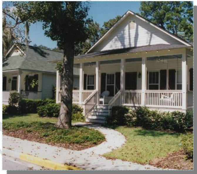
Example of Single-Family Residential--Sewered
