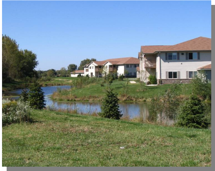
Stormwater Facility for Multi-family Residential
