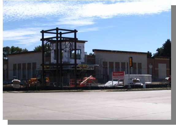
New Walgreens on redevelopment site
